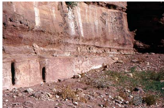
Water Management in Petra. Fig. 6 Dual pipelines continuing past the theater to supply tanks (T) above the Cardo.
